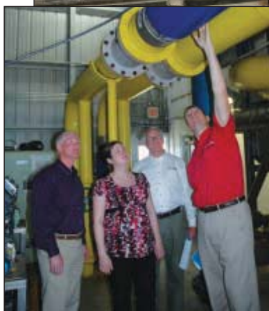
Clean Water Award judges inspect sludge bulk conditioner on DAF feed pipe.
