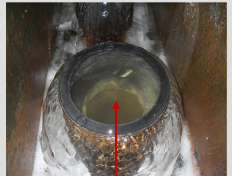
EDGE Effluent with Organic Coagulant
