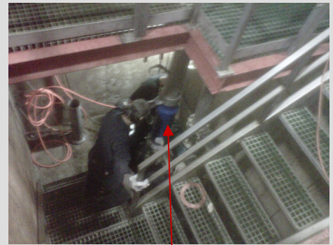
Installing EDGE Reaction Chamber
